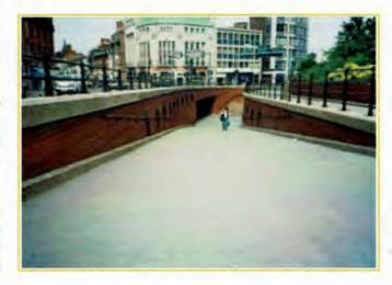
A clear or coloured seal coat can be applied to the surface to maintain its visual appearance and to make it easier to clean.
